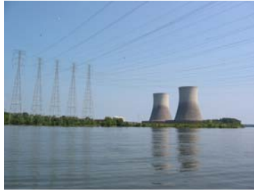
Sequoyah nuclear power plant
